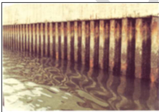
Photo 2.7.7 Corrosion conditions ( ii )
