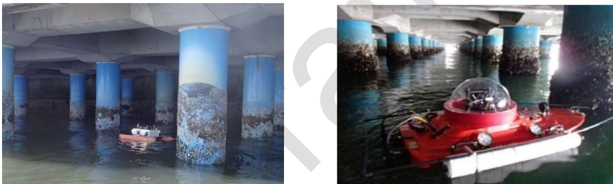
Photo 2.2.5 Survey of the underside of the pier using an ROV and a small radio boat
