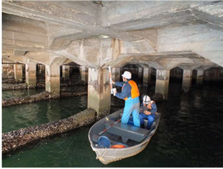
Photo 2.2.1 Visual inspection of a wharf superstructure
