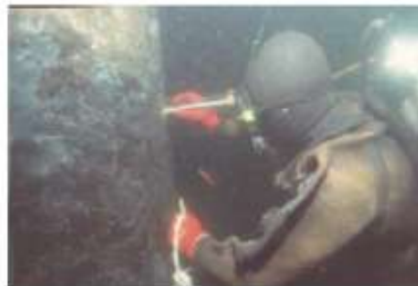
Photo2.2.2 Visual Inspection of the Underwater of Steel Sheet Piles
