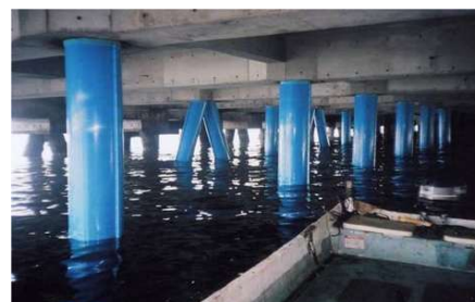
☒ 2.7.1 An Example of Corrosion Protection Method applied to Open-type Wharf
