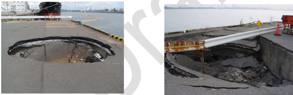
Photo 2.4.1 Example of hole in apron caused by cavity
