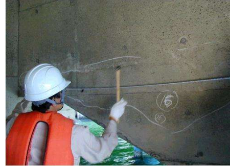
Photo 2.2.1 Visual inspection of a wharf superstructure
