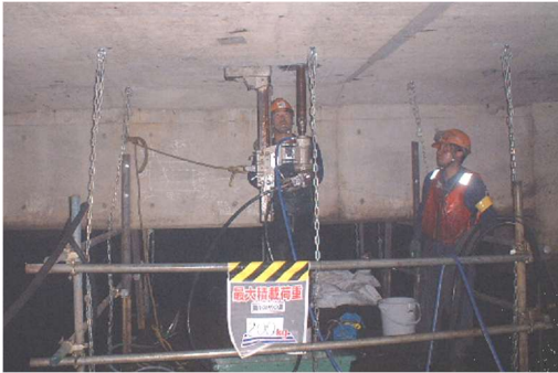
Photo2.6.4 Core sampling status and depth-sliced core samples
